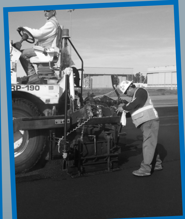
Mini-Line® HS301 Grade Control Kit with G221
